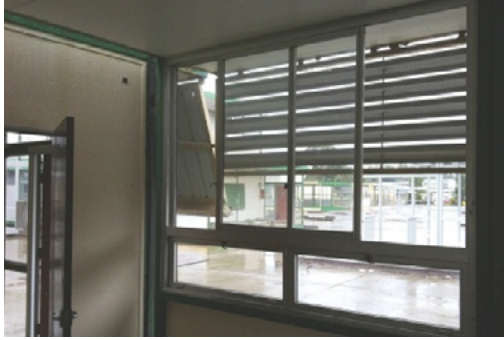
Photograph 05: Typical windows – view from inside demountable
