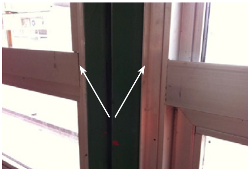
Photograph 06: Position where asbestos containing mastic is used to seal the join between the steel frame of the demountable and the aluminium frame of the windows / panels
