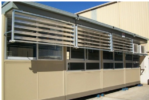
Photograph 02: Old system demountable showing typical wall panels and windows – view from rear
